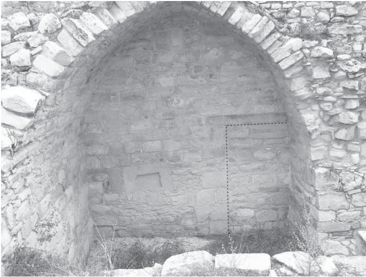
Fig. 65: Pano Polemidia, Karmiotissa, sealed doorway at the eastern end of the north wall [M. Olympios].
